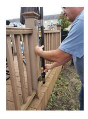
9) Slide the pole through the attached upper Deckhands<sup>™</sup> clamp and replace the lower Deckhands<sup>™</sup> clamp on the pole. Adjust to the desired installation position. Use a level to ensure the pole is vertical. Mark the round hole locations on the lower Deckhand<sup>™</sup> clamp.
