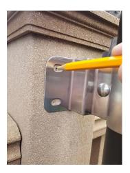
13) Mark the hole locations for the slot side of the upper and lower Deckhands™ clamps. The location should be toward the outer edge of the slot. The clamp should be in the tightened position.
