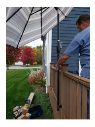
19) Loosen both Deckhands™ clamps knobs and adjust umbrella height and rotation as needed keeping in mind the tilting position of the umbrella for optimal shading. Hold the umbrella securely while both Deckhands™ clamp knobs are loose.
