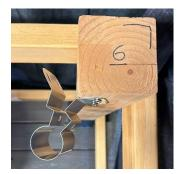
Carefully screw in the screws in the holes, do not fully tighten. Leave loose enough to move the Deckhands<sup>™</sup> clamp.
