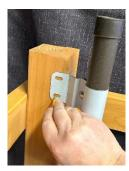
3) Hold the pole with the attached Deckhands<sup>™</sup> clamps against the corner support in the desired position. Adjust the positioning of the Deckhands<sup>™</sup> clamps as desired. Mark the location of the holes. Holes should be toward the outer edge of the slots. The Deckhands<sup>™</sup> clamps should be in the tightened position. Hold still while marking the holes in the top and the bottom.
