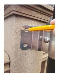
13) Mark the hole locations for the slot side of the upper and lower Deckhands<sup>™</sup> clamps. The location should be toward the outer edge of the slot. The clamp should be in the tightened position.
