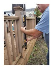
9) Slide the pole through the attached upper Deckhands<sup>™</sup> clamp and replace the lower Deckhands<sup>™</sup> clamp on the pole. Adjust to the desired installation position. Use a level to ensure the pole is vertical. Mark the round hole locations on the lower Deckhand<sup>™</sup> clamp.
