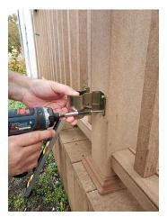
11) Install the screws the same as the upper. Leave the screws slightly loose.
