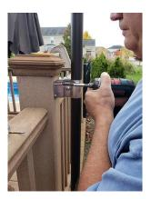
15) Install the screws in the slot holes as done for the round holes. Leave slightly loose. Do for both upper and lower.
